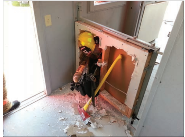
A course Instructor breaches a wall in the Firefighter Skills trainer during a train-the-trainer for the Firefighter Skills training course.
