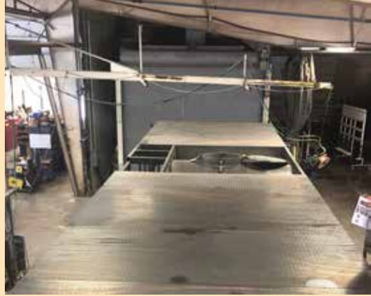
The tank prop and hatch under construction (top view of trailer)
