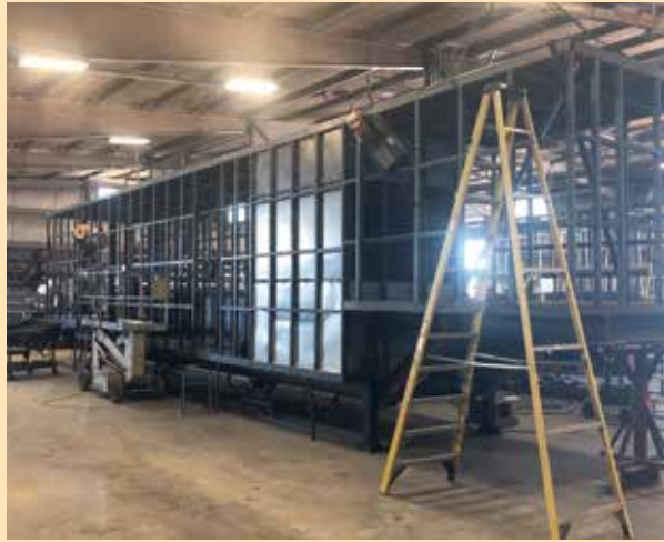
Confined Space Trainer under construction at Unruh Fire in Sedgwick, KS.
